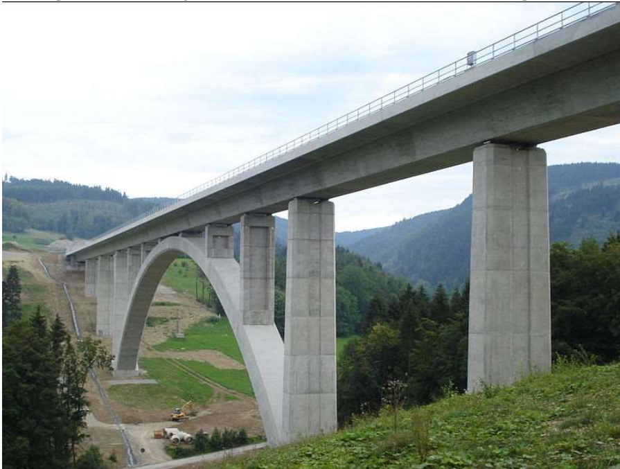
Bridges erected by ILM – SOFiSTiK: Trunkenthalbridge, Germany
